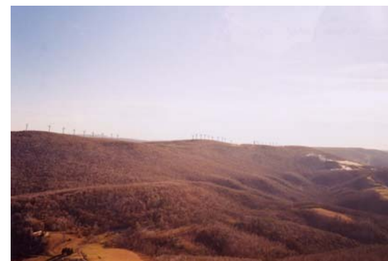
The 65-MW Backbone Wind Farm On-Line September 2003
