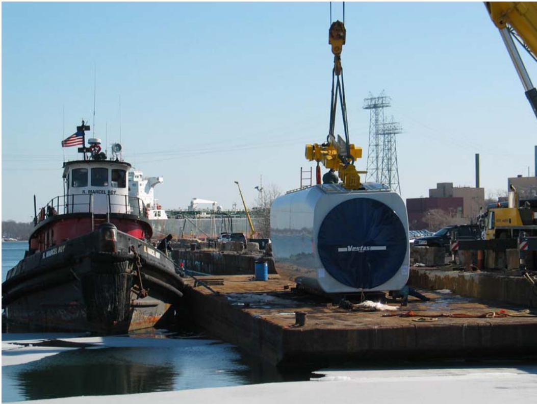
Figure 14 Nacelle Arriving in Quincy Harbor (Photo: Mark Brennan)
