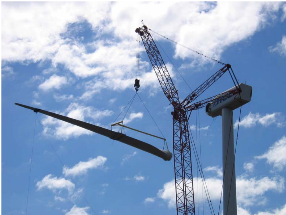
Figure 18 First Blade Installation
