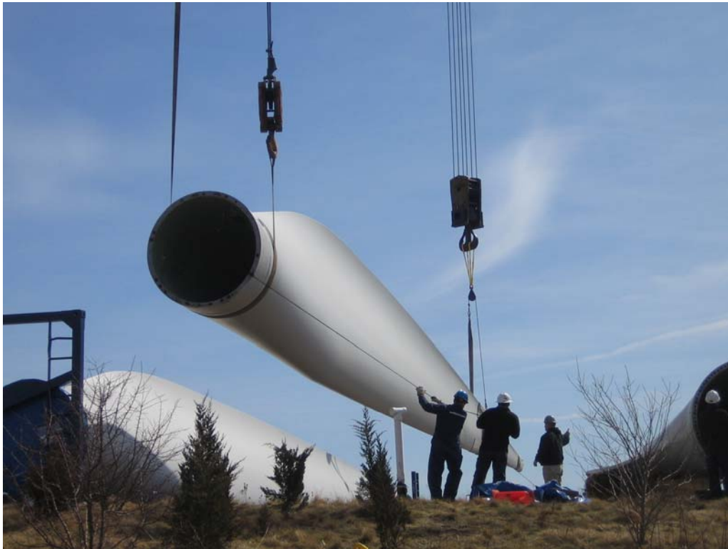
Figure 17 Blade Lifting Process
