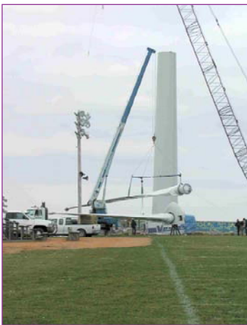
Assembly of Hull Wind One's rotor
