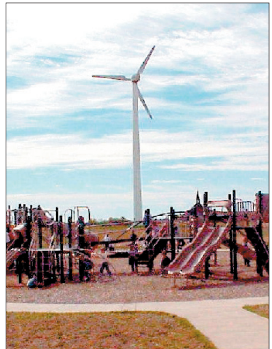
Community-owned wind turbine in Spirit Lake, IA
