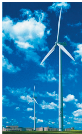
Community-owned 750 kW wind turbine in Moorhead, Minnesota.
