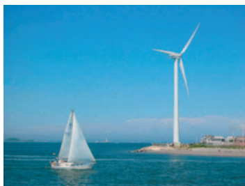
Community-owned wind turbine in Hull, MA.
