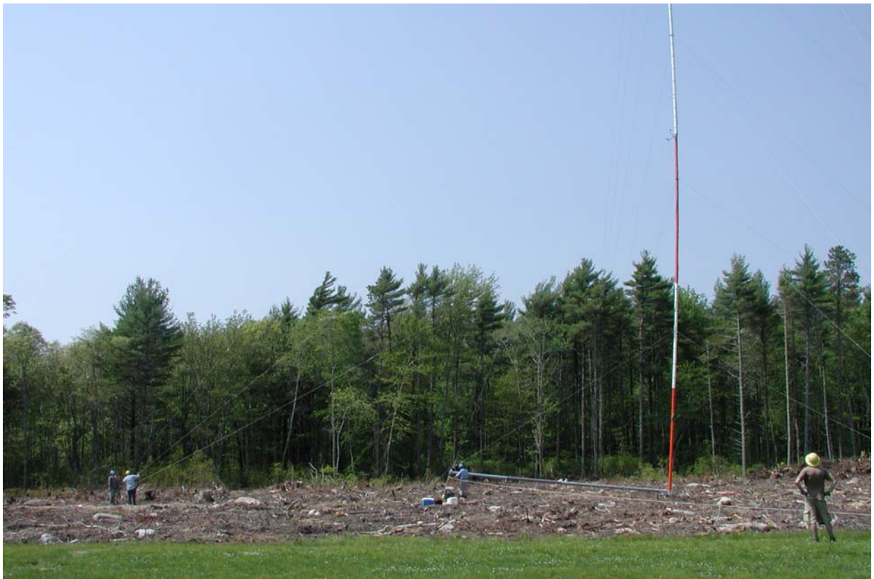
Figure 2 – Raising the Met-tower at ORR Site
