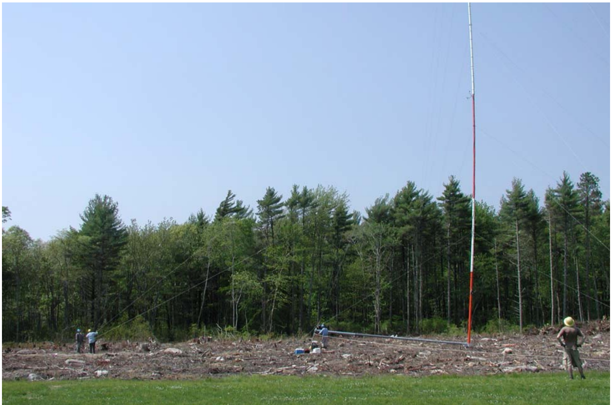
Figure 2 – Raising the Met-tower at ORR Site
