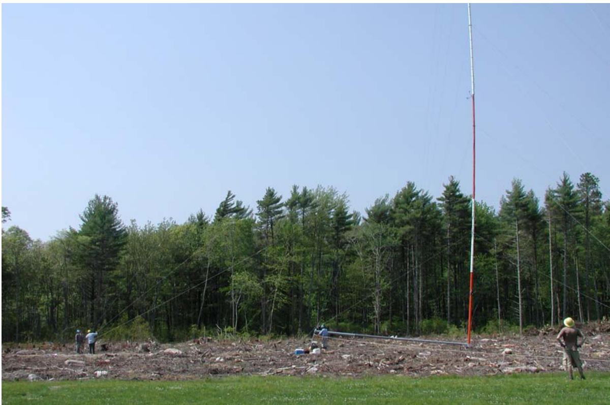
Figure 2 – Raising the Met-tower at ORR Site
