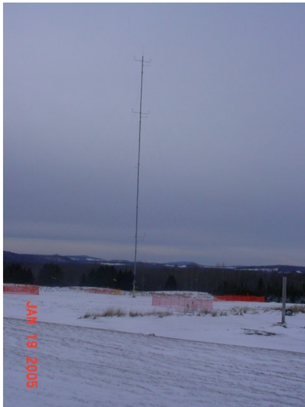
Figure 2 – 50 m data tower in Presque Isle soon after installation.
