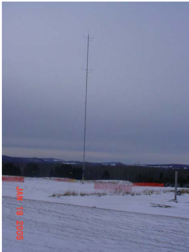
Figure 2 – 40 m data tower in Presque Isle soon after installation.
