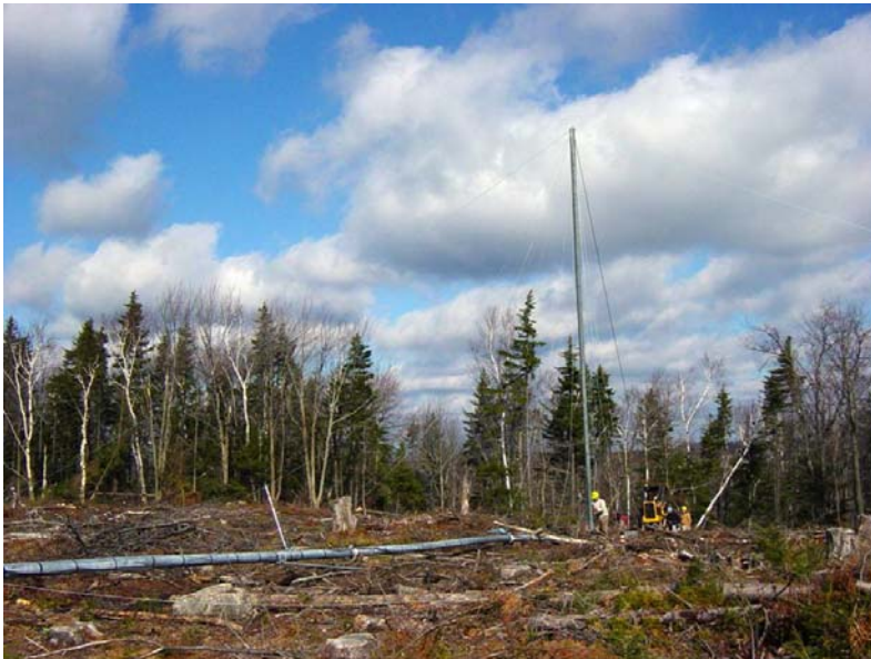
Figure 2 – 50m data tower in Savoy during installation.
